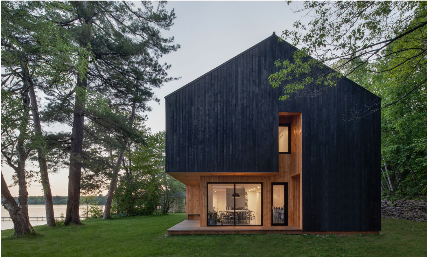
This house was designed by the Canadian architecture studio Schwimmer and is located East of Montreal, near lake Brome. The architects used charred wood, a technique from Japan that is increasingly more popular, namely because it reinforces the coating's waterproofing and repels insects.
